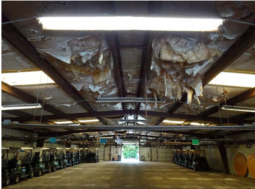
Photo (2021) of damaged insulation in the cart barn, an example of improvement needs to this facility.
