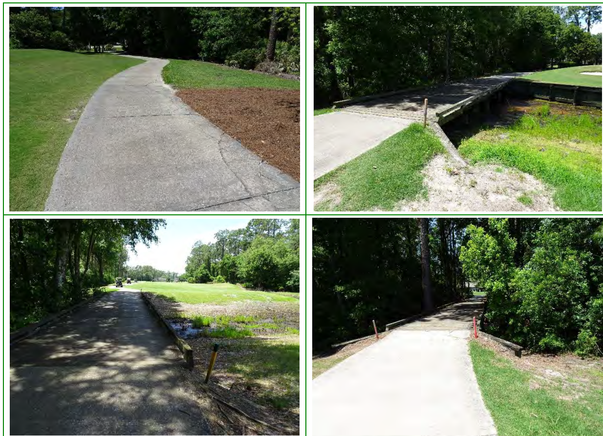
Images (2021) of EHGC cart paths and bridges showing some areas of cracking and surface damage that should be addressed.
