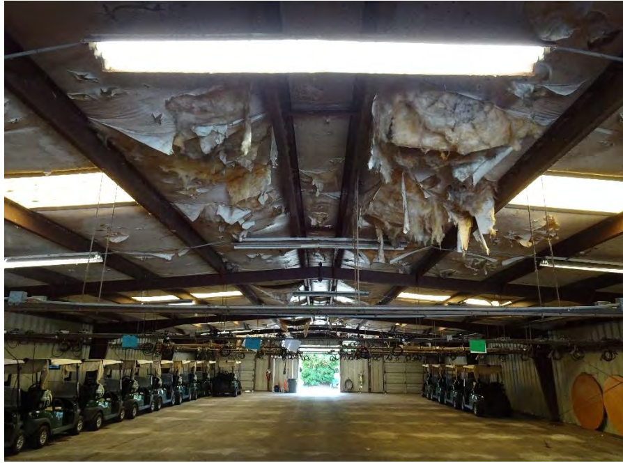
Photo of damaged insulation in the cart barn, an example of improvement needs to this facility.
