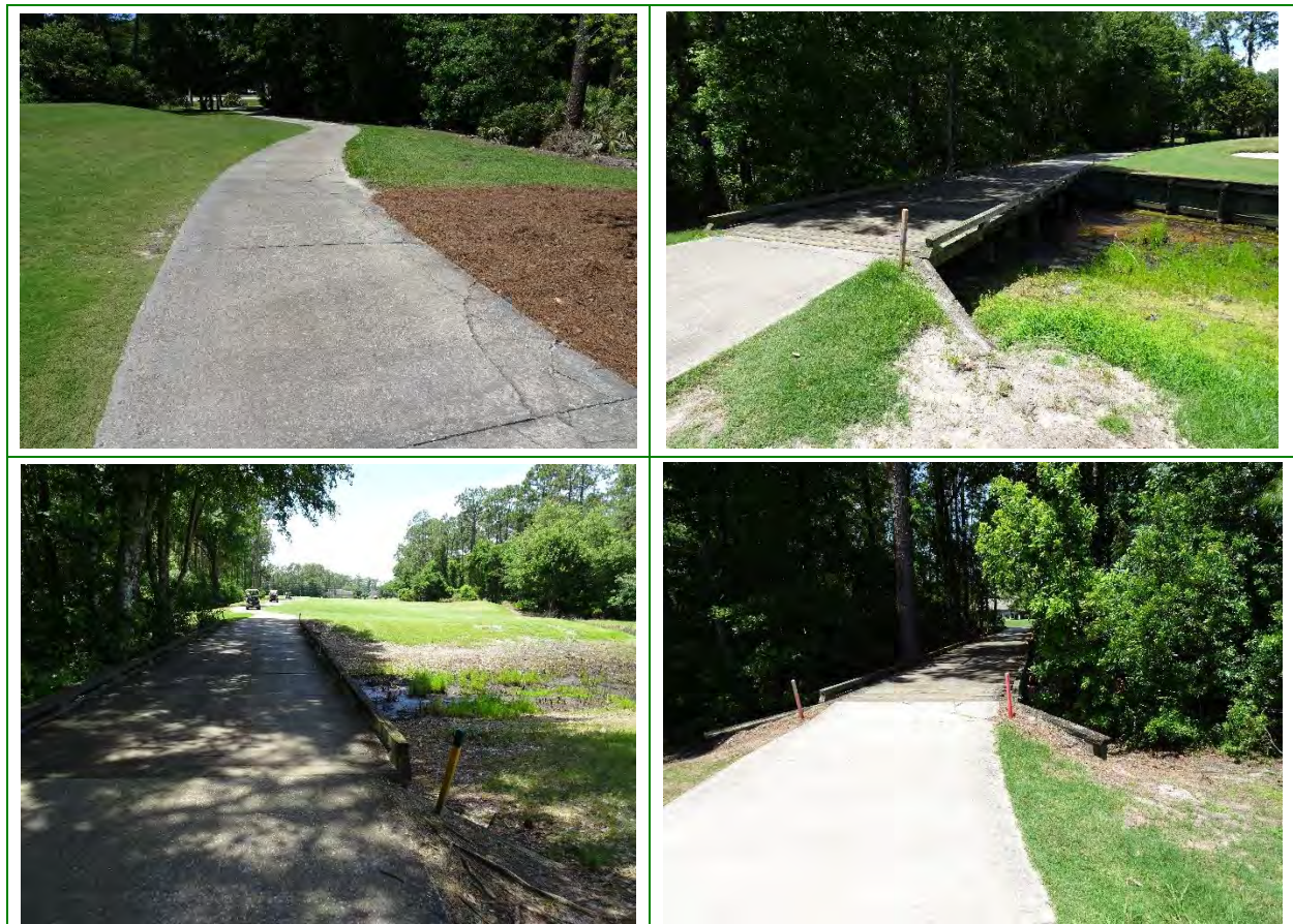
Images of EHGC cart paths and bridges showing some areas of cracking and surface damage that should be addressed.
